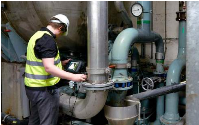
Industrial pipeline inspection with Proceq Flaw Detector 100
