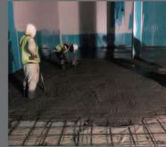
Concrete Flooring & BRC Laying
