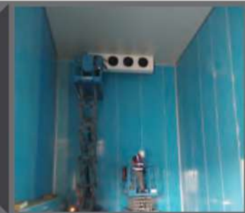
Evaporator / Blower Installation
