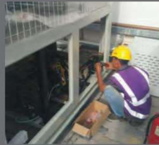
CDU & System Assembling Works
