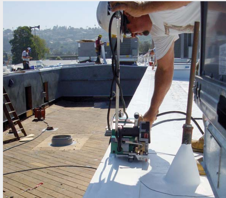
Its small dimensions mean that there are no obstacles for the UNIROOF E.
