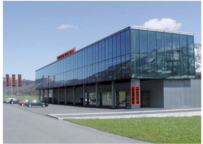
Leister Corporate Center in Kaegiswil, Switzerland.
